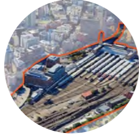
04. Railway Square Redevelopment
