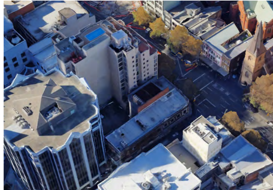
Above: Current Condition, Google Images
