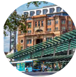
03. Railway Square Bus Terminal
