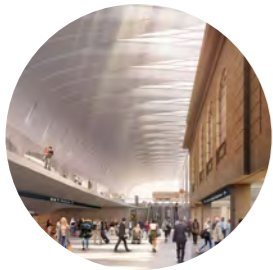
01. Central Station Redevelopment
